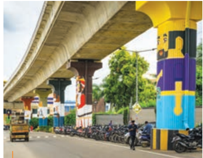
Pier wall painting at the Biocon-Hebbagodi Metro station
