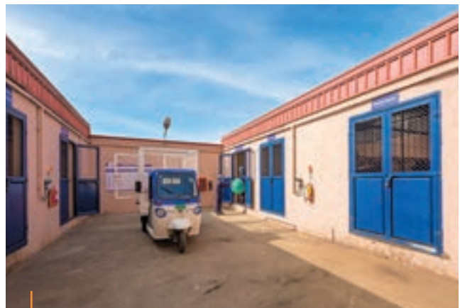
Waste segregation system at Biocon Park, Bangalore
